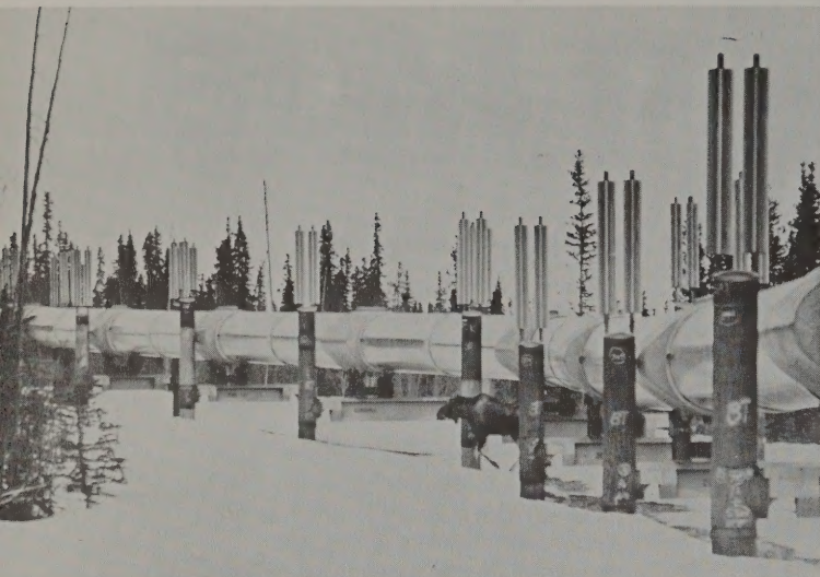
A moose passes beneath a section of above-ground pipeline. Animal crossing places are provided frequently along the pipeline.
